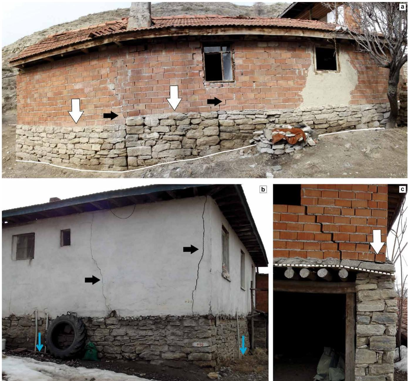
Figure 4. (a) Displacement of house wall showing bulging and cracking caused by subsidence, and broken windows due to distortion. (b) Cracks on wall and pipes draining wastewater directly into ground. (c) Open joint in wall of building. (Photographs taken on February 26, 2017).
